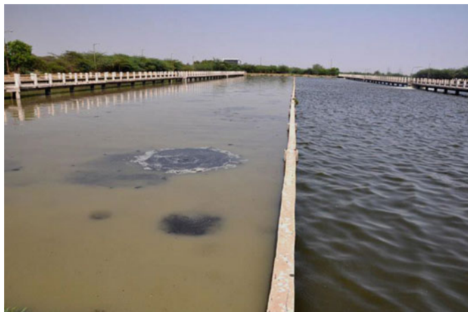
Fig. 2 Anaerobic waste-water treatment by sludge upwelling followed by Rhodospseudomonas stage (In Karnataka, India. Unpublished data)
