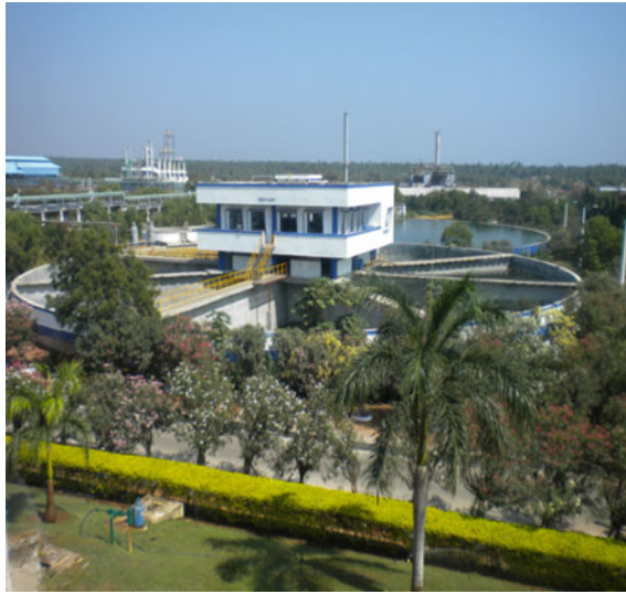
Fig. 22 Guard pond complex
