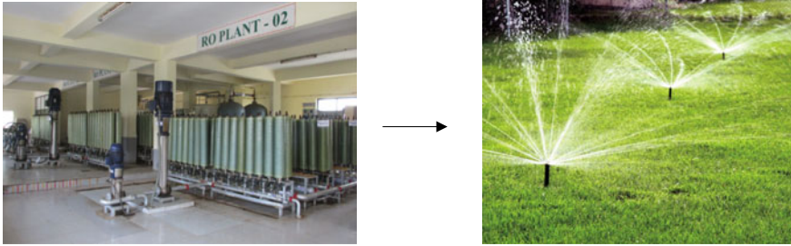
Fig. 9 Reverse osmosis plant, rejected RO water used for plantation
