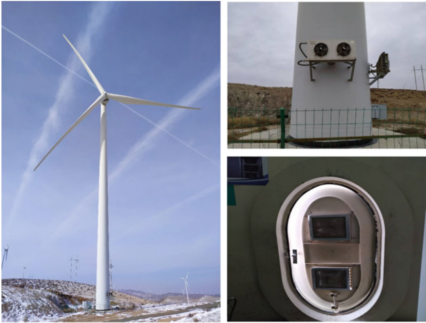
Fig. 1 Wind turbine tower
