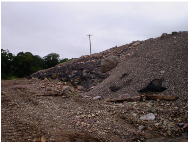
Fig. 2 Construction of anti-deformation measures of the railway embankment on thawing permafrost
