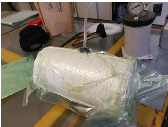
Fig. 3 FRP confinement by using in-fusion process
