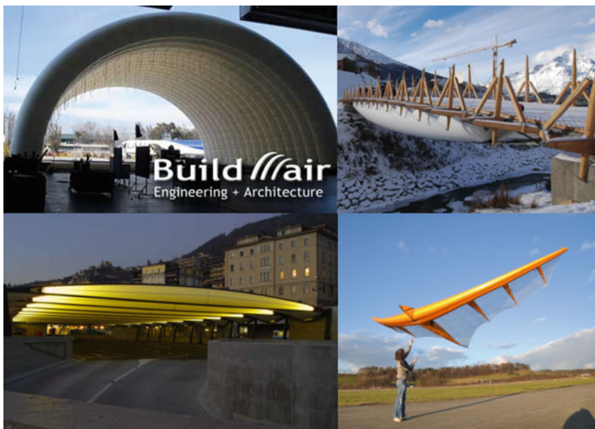
Fig. 6 Tensairity has already been applied successfully as long span beams on a roof and on a bridge, portable hangars and kites [12, 14]
