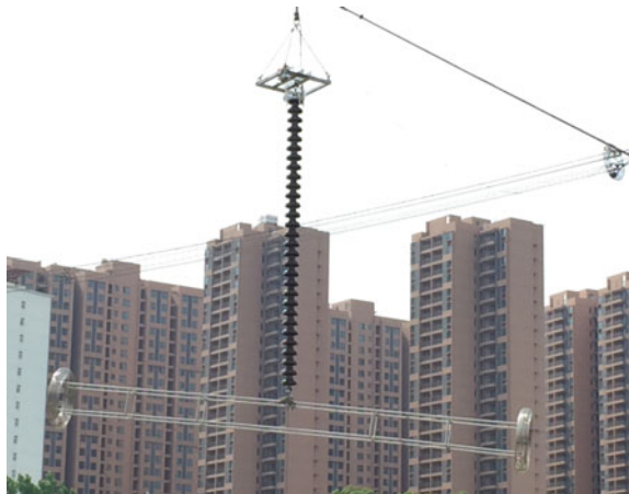
Fig. 12 Test platform of the insulators string
