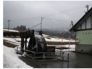
Micro hydro electricity test equipment
