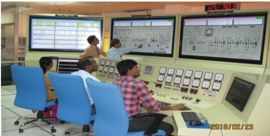
Fig. 8 Development work in progress
