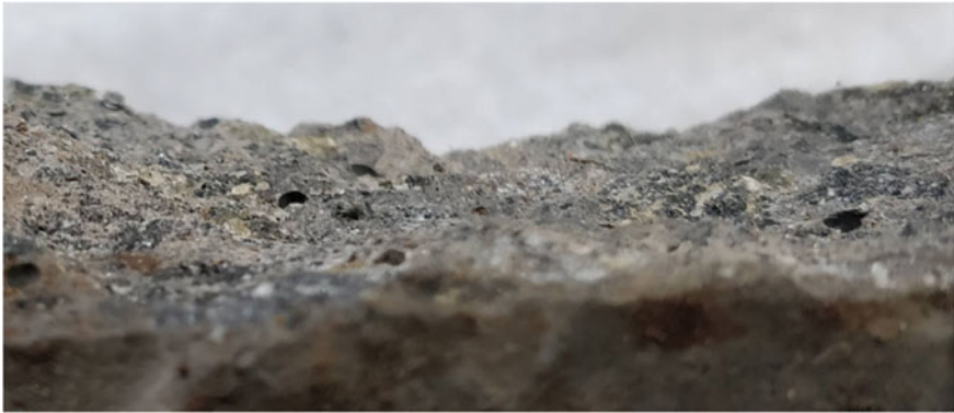
Fig. 9 Fractured surface of conventional concrete beams
