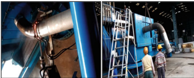
Fig. 9 70° trial bend during bending and unloading
