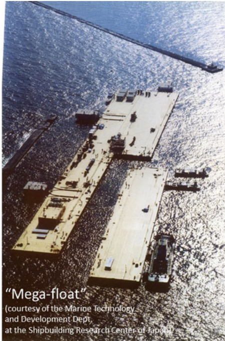
Fig. 2 Photograph of “Mega-float”
