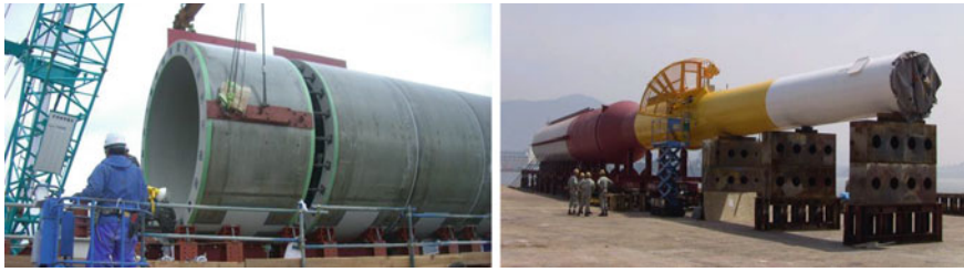
Fig. 4 Assembly at quay yard
