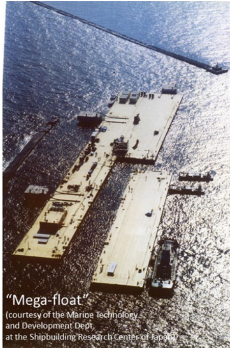
Fig. 2 Photograph of “Mega-float”
