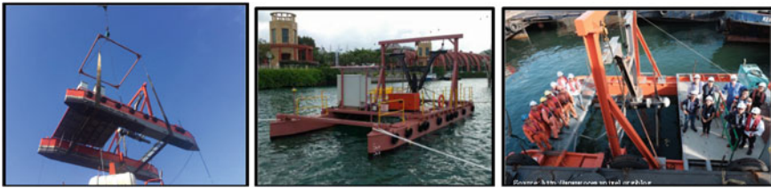
Fig. 28 Fully fabricated tidal energy system in Singapore
