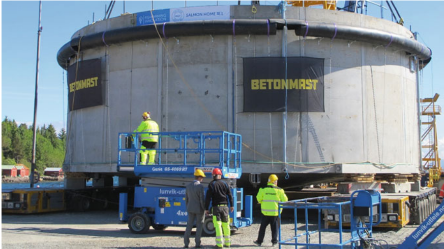
Fig. 21 Completed bucket ready for lift out
