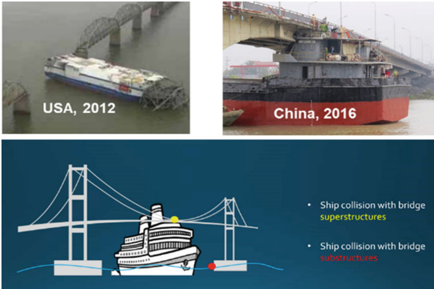
Fig. 11 Ships have impacted bridges. Ships might hit pontoons or superstructures of floating bridges (Courtesy: Dr. Yanyan Sha, NTNU)
