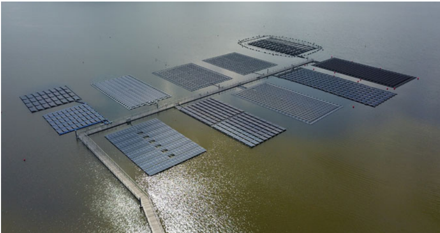
Fig. 5 The 1MW p floating solar testbed at Singapore's Tengeh Reservoir (Source SERIS)
