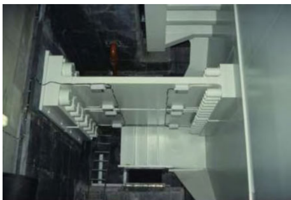
Fig. 7 Flexible plates, 3.5 m long and 126 mm thick, connecting the bridge girder of the Nordhordland FB to its abutment [5]
