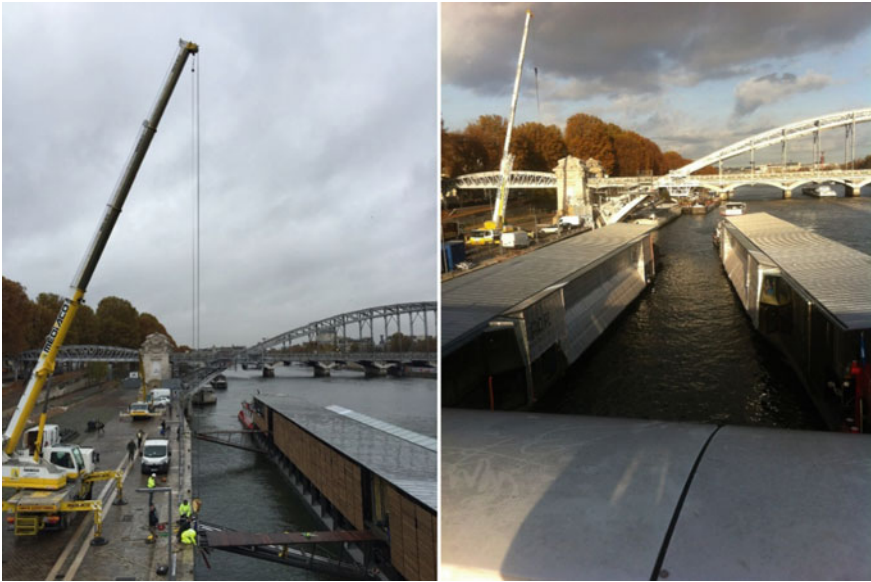
Fig. 13 Final assembly of two hulls and connections to the shore
