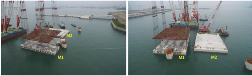
Fig. 15 Main module connections
