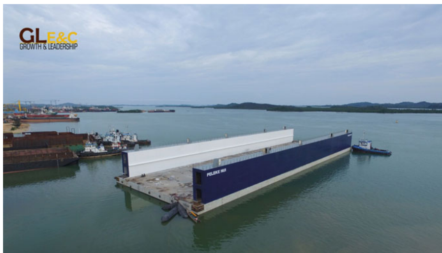
Fig. 5 Completed concrete dry-dock 1st May 2017
