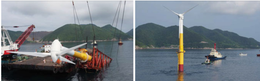
Fig. 5 Installation of the half-scale model
