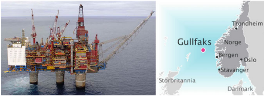
Fig. 3 Gullfaks C, its final destination, built in, and transported from Stavanger
