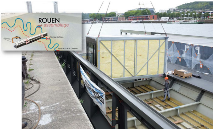
Fig. 12 Installation of modular superstructure
