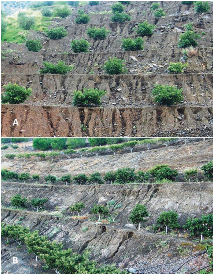
Fig. 7.2 Rills and gullies in the taluses of avocado (a), mango and loquat (b) orchard terraces after a heavy rainfall event
