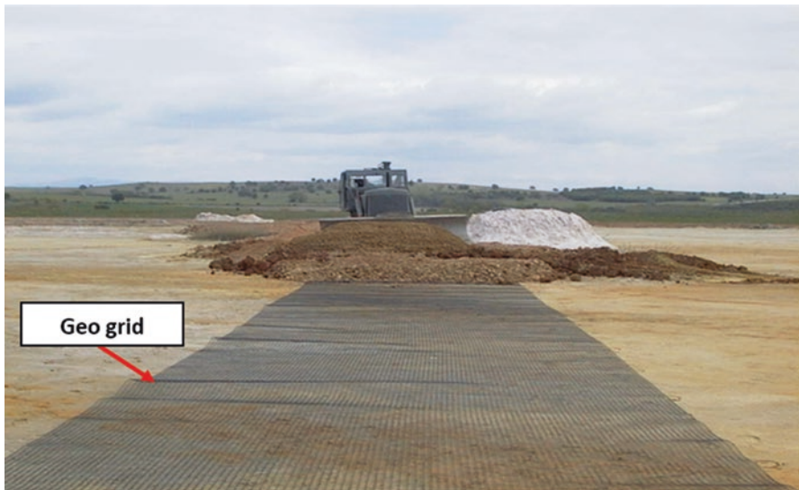
Construction of temporary roads
