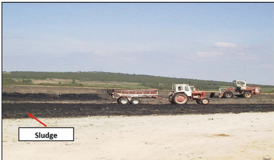
Spreading of stabilized sludge from the Plovdiv wastewater treatment plant
