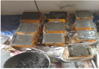
Fig. 1. Casting of concrete
