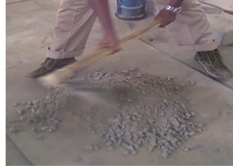
Fig. 2. Mixing of concrete
