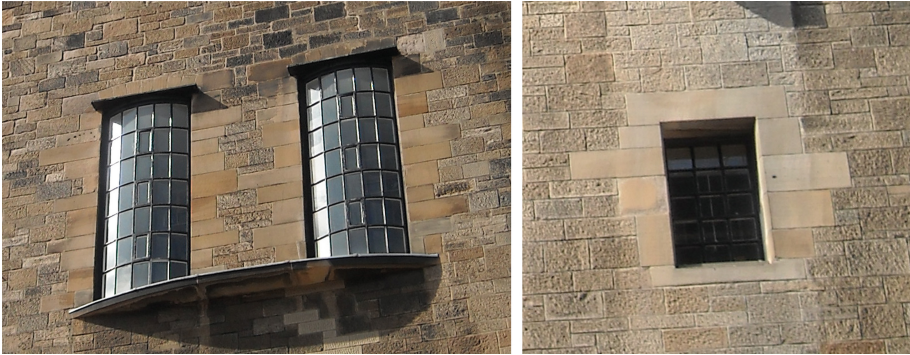
Fig. 7. Photos of two windows of the East Façade of the Glasgow School of Art. Around the windows, it is possible to recognize the ashlar. The photos also show the variation of the stone color (Source: Personal archive of the author).
