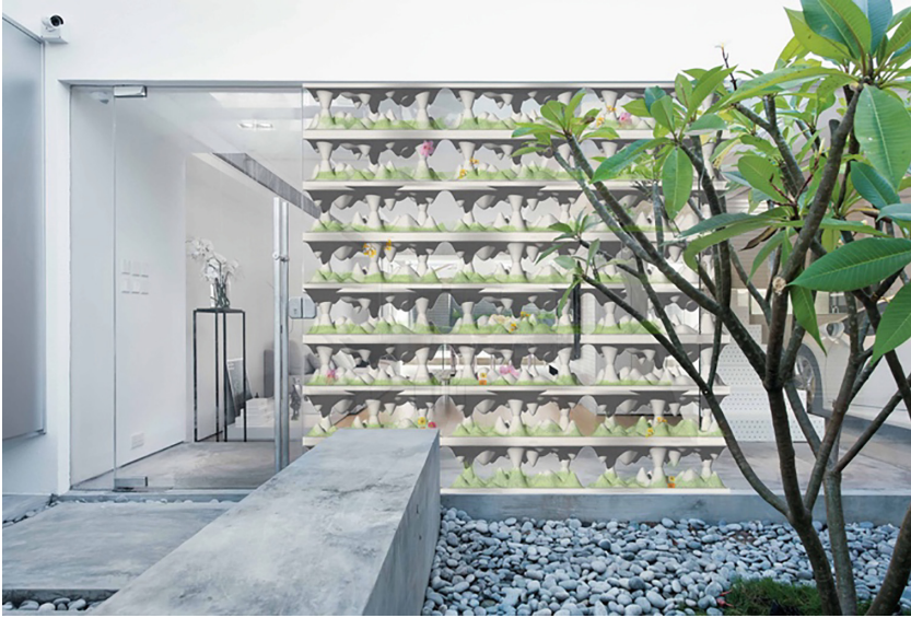
Fig. 7. Application of weeping brick to living wall brick system
