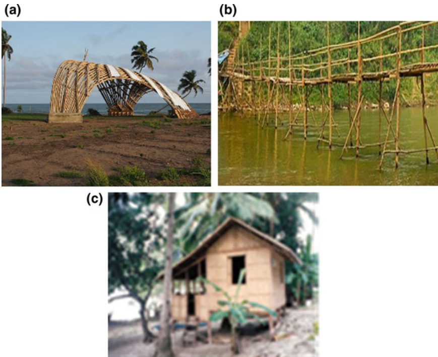
Fig. 2 a Bamboo canopy structure for realisation, b Bamboo walking Bridge, c Bamboo Houses. Source [20, 21]
