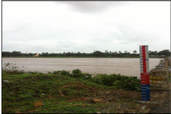
Fig. 6 Flood level indicator
