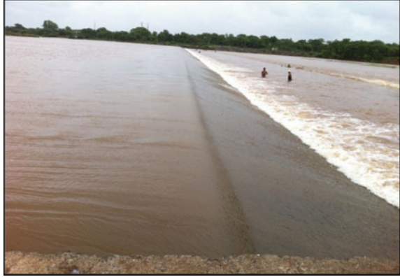
Fig. 4 D/S side of Ambica river
