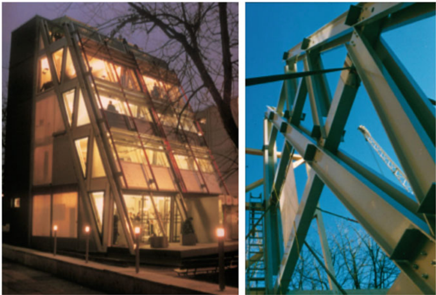
Fig. 3 Eyecatcher building, Basel, 1998: three load-bearing frames, bolted joints [35]
