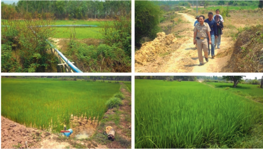
Fig. 1 Piping irrigation system completely constructed in Bungmalang sub-district, Sawangweerawong district, Ubon Ratchathani province, 2009
