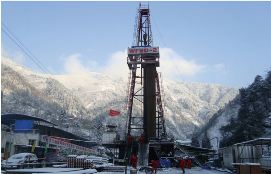
Fig. 3.4 Site of the WFSO-2 borehole
