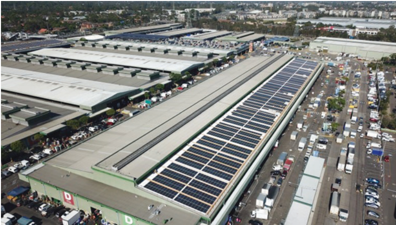
Fig. 3.6 View of part of the 2.2 MW PV rooftop system on Sydney Markets (Source Autonomous Energy (used with permission of Matthew Linney))
