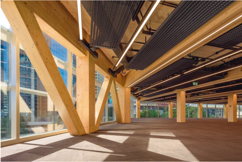
Fig. 9.5 International House, Barangaroo. Timber as a low carbon structural material in multistorey commercial buildings ( Source Tzannes Associates, with permission)
