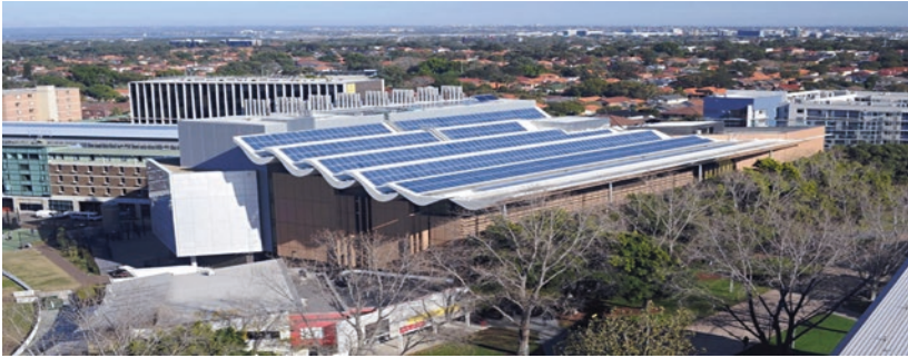
Fig. 3.4 Tyree Energy Technology Building, UNSW 6 star Greenstar building with a 150 kWp PV array (Source School of Photovoltaic and Renewable Energy Engineering, UNSW)
