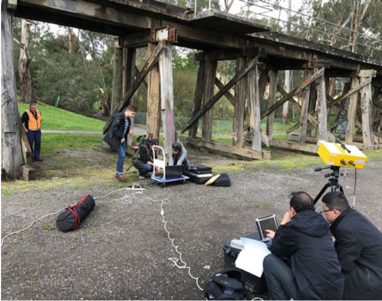
Fig. 1 Structural monitoring of the bridge using IBIS-S and ARAMIS
