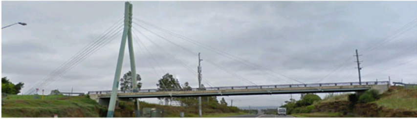
(a) The cable-stayed bridge
