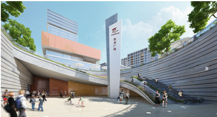
Fig. 5. Metro Huijin Road Station Exit 2 docking Baolong Square
