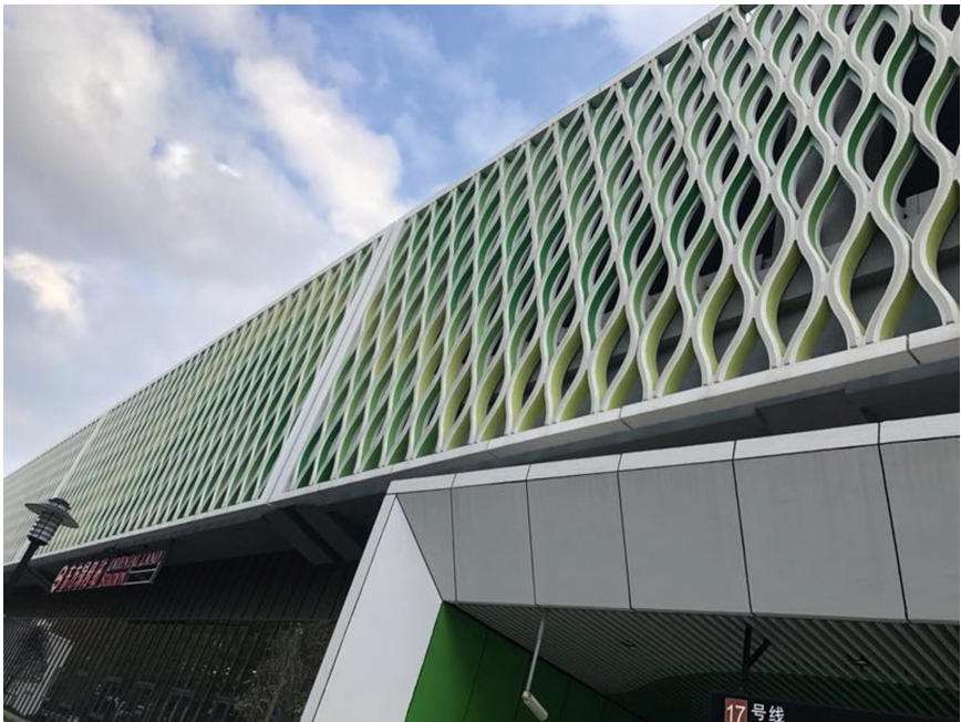
Fig. 7. Application of PC technology in Oriental Green Boat Station
