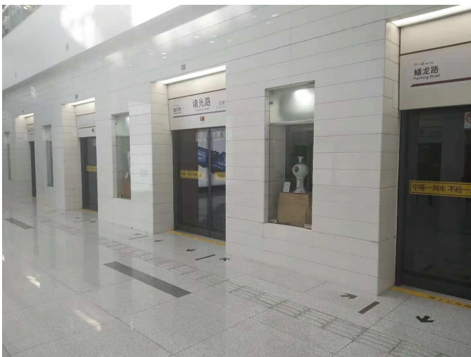
Fig. 2. Zhuguang road station
