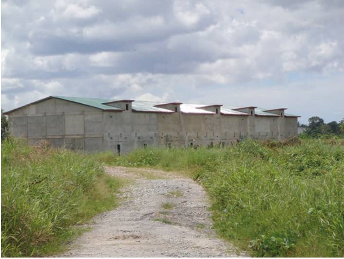
Fig. 20.10 The appearance of a swiftlet house in Asajaya is similar to a longhouse. (Photograph: Tetsu Ichikawa 2011)
