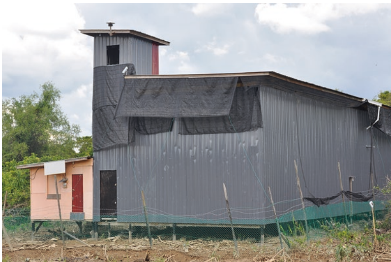
Fig. 18.1 Swiftlet house in Daro. (Photograph: Daniel Chew 2012)
