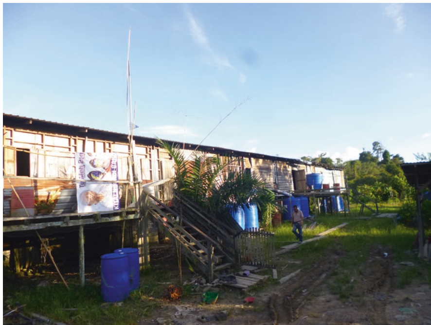
Fig. 15.9 Exterior of a longhouse in AB village. (Photograph: Ryoji Soda 2013)
