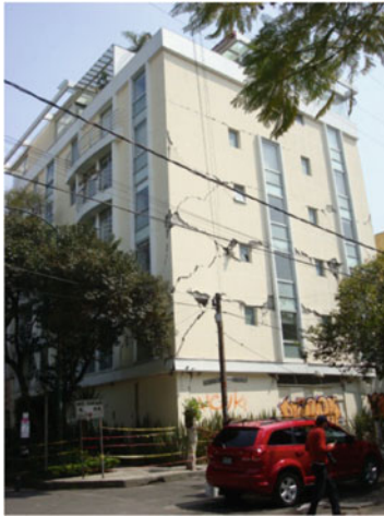
(a) 6-story building
