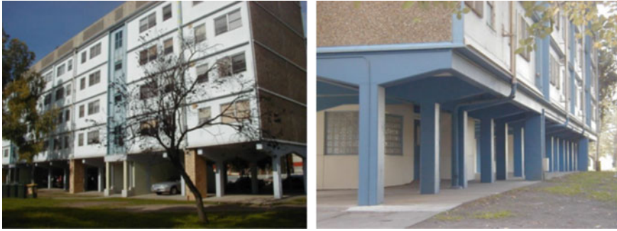
Fig. 3 Typical soft-storey buildings (photos taken by Hing-Ho Tsang)
