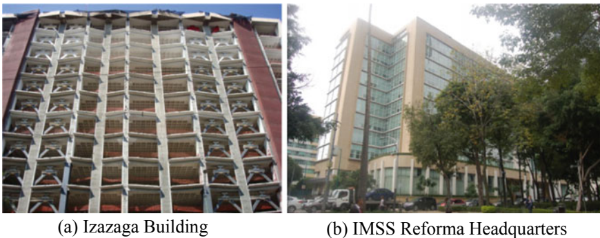
Fig. 6 Pictures taken shortly after the September 19, 2017 earthquake for two office buildings in Mexico City retrofitted during the 1990s with ADAS energy dissipation devices as structural fuses. The buildings survived the earthquake with no damage
