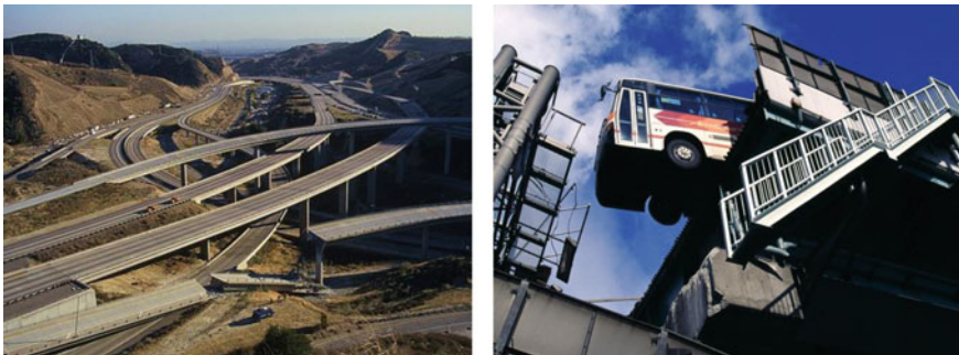
Fig. 24 Damage of motorway bridges during the 1994 Northridge earthquake (left); and a bus marginally stopping before a collapsed bridge of Hanshin Expressway Route No. 3 (right)
