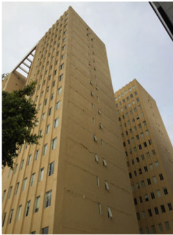
(a) 17-story building
