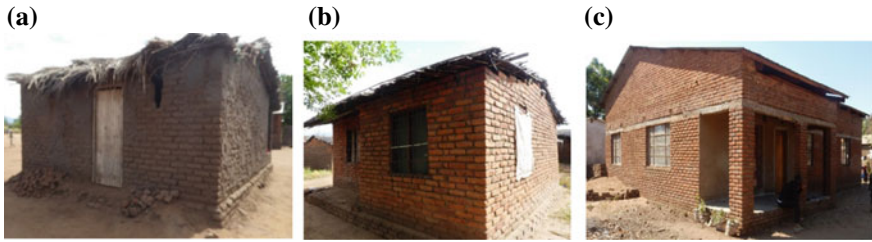
Fig. 5 Typical one-storey masonry building in Malawi. a typology A; b typology B; c typology C
