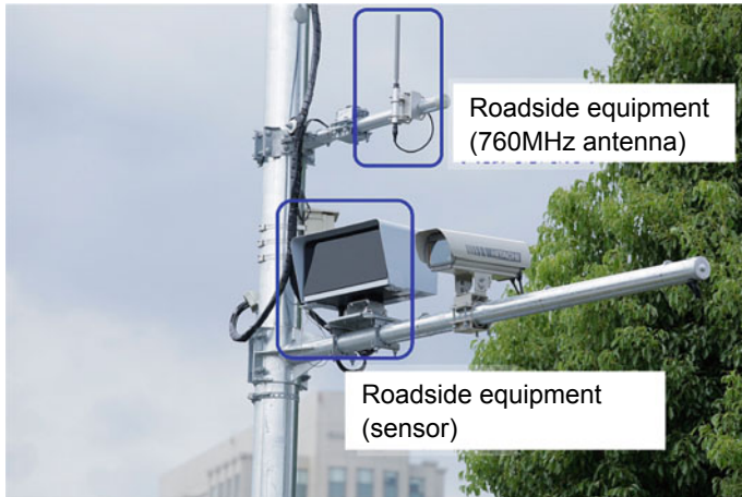
Fig. 5 An antenna of vehicle-to-infrastructure communication with 760 MHz and a sensor
