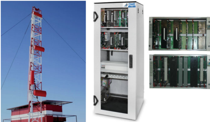
Fig. 4.34 Antenna system and the box for GP734 with DME734. Source http://www.nports.ru/#!/catalog by permission of LLC Research and development company “Radio engineering systems”
