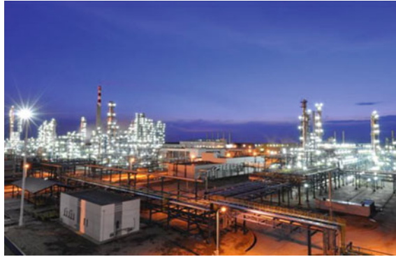
Fig. 3. Oil field refinery
