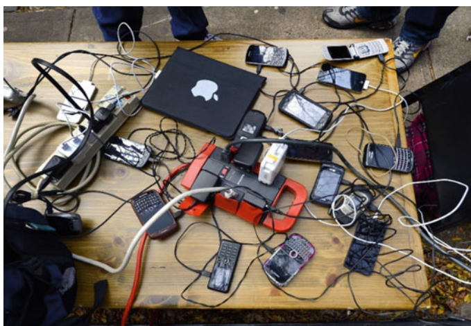
Fig. 4 A wired mess consisting of charging wires
