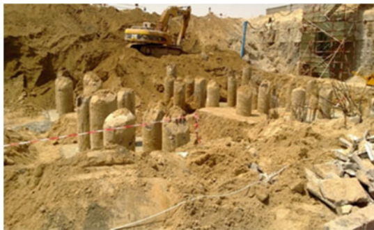
Fig. 1 CFA piles underneath the current building in UAE
