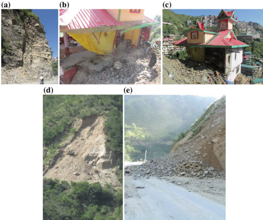
Fig. 9 a Rock slide occurred along the NH 5A in Shimla town. b and c settlements damaged due to the landslide. d and e landslide occurred along a place called Luhri located in Shimla—Rampur National Highway
