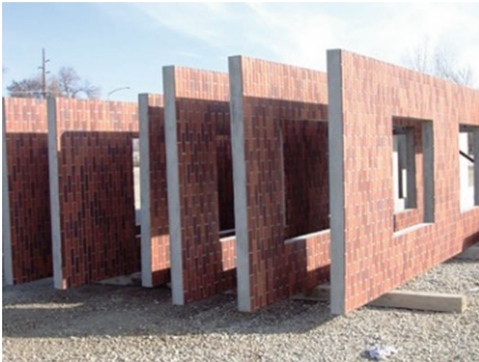
Fig. 6 Pre cast walls
