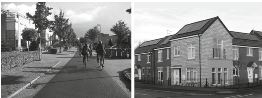
Fig. 2.2 Housing estates designs to incorporate environmental and social-friendly elements such as cycling, roof tops with solar panels. Source Falk and Carley (2012), and author
