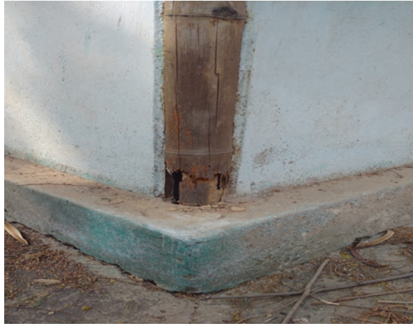
Fig. 6 Decay of untreated bamboo (IIT Delhi, India) in about 5 years of installation
