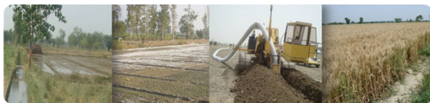
Fig. 1 Soil condition before and after installation of SSD. Source CSSRI Annual Report
