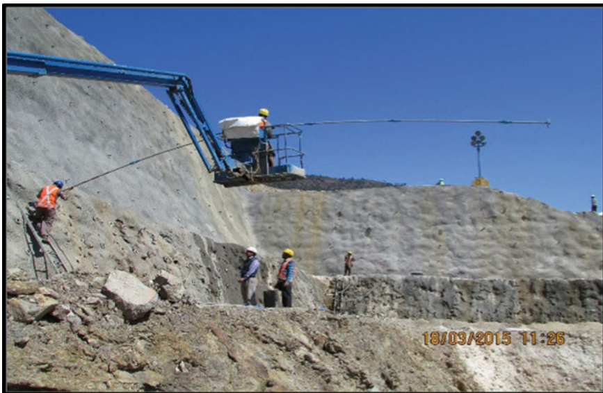
Fig. 18 Installation of rock bolts in progress
