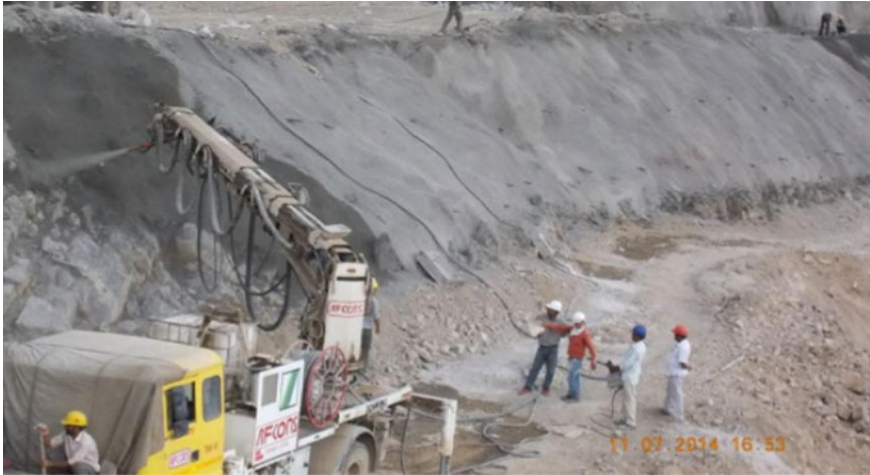
Fig. 17 Application of 50 mm thick steel fibre-reinforced shotcrete
