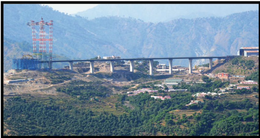
Fig. 3 Completed viaduct on the right bank
