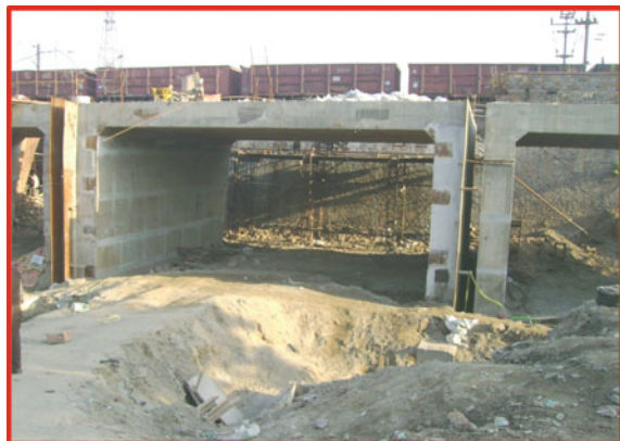
Fig. 7 Construction of boxes
