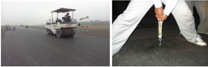
Fig. 4 Rolling and adhesive testing of glass grid
