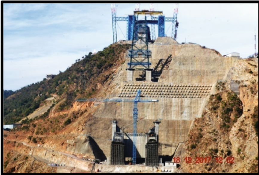
Fig. 6 Stabilized slopes on the right bank
