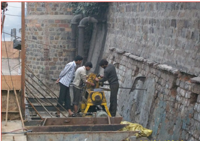
Fig. 3 Installation of test nail
