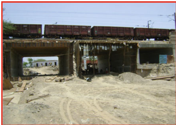
Fig. 13 GI sheet installation
