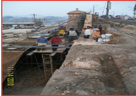
Fig. 9 Dismantling of wall
