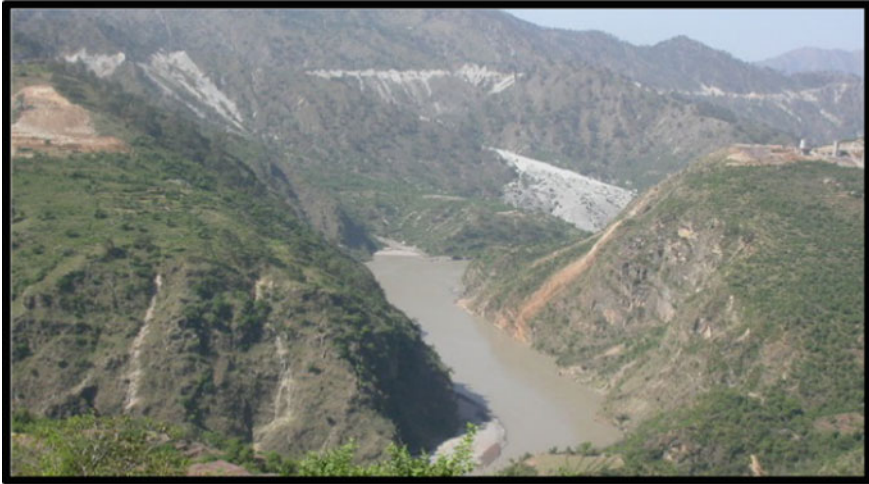
Fig. 2 Left and right banks of Chenab Bridge before commencement of work
