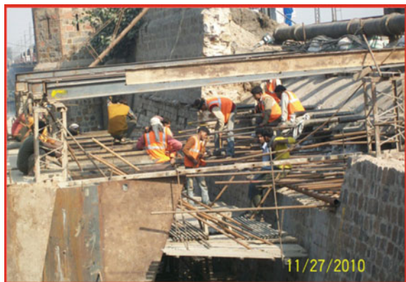
Fig. 8 Installation of girder
