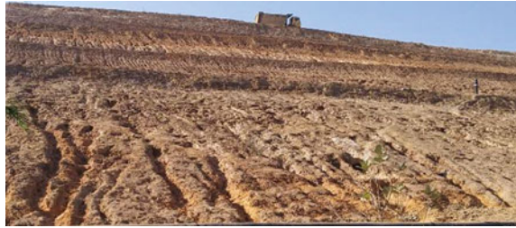
Fig. 2 Typical view of jarofix mound at Chittorgarh
