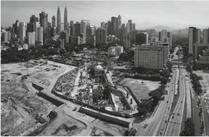
Fig. 12 Ariel photo of Tun Razak Exchange station in construction, after rock fissure grouting
