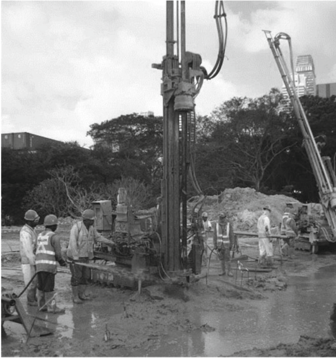
Fig. 16 Triple-fluid jet grouting
