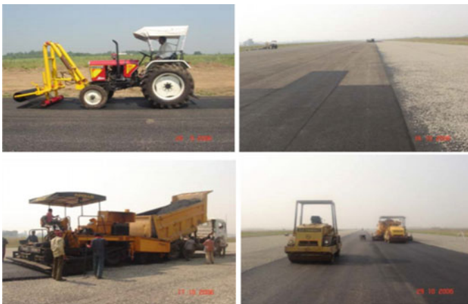
Fig. 5 Laying of glass grid, SAMI, and DBM
