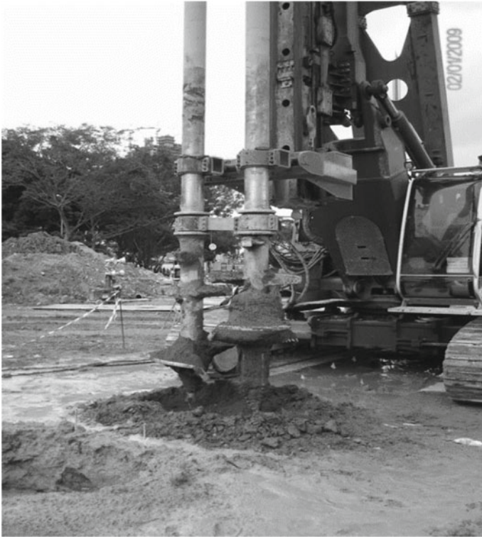
Fig. 15 Deep soil mixing rig with overlapping twin paddles
