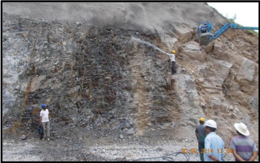
Fig. 15 Cleaning of excavated slope with water jet
