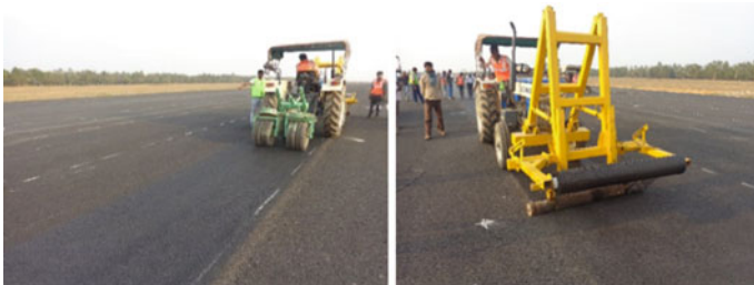
Fig. 3 Laying of glass grid
