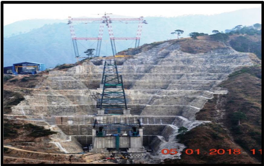
Fig. 5 Stabilized slopes on the left bank
