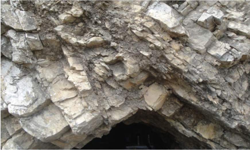
Fig. 7 Rock mass exposed at the bridge site
