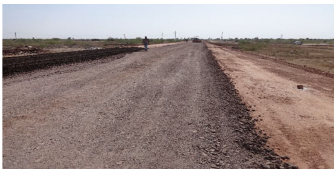
Fig. 8 Prepared CTSB surface
