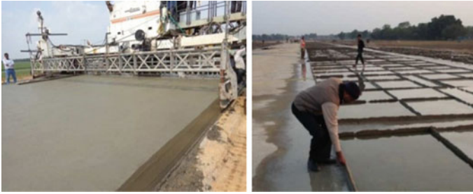
Fig. 6 Laying of PQC
