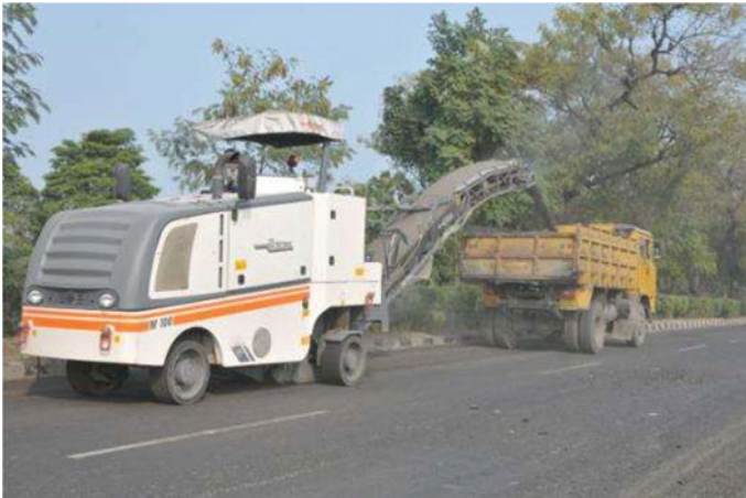
Fig. 11 Milling of the existing bituminous surface for RAP material
