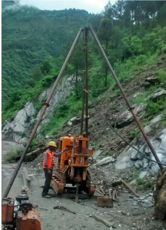
Fig. 4 Borehole drilling in progress—Note the slide material on the hillslope
