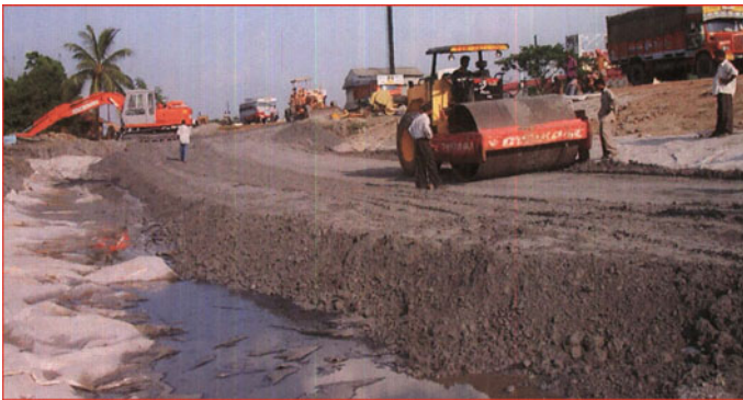
Fig. 6 Four laning work of NH 6 from Dankuni to Kolaghat
