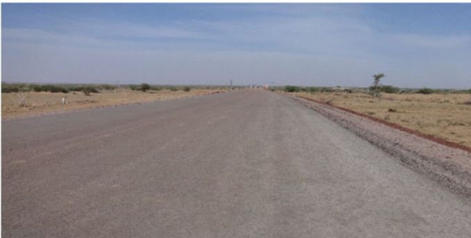
Fig. 16 Finished foam bitumen-treated RAP surface
