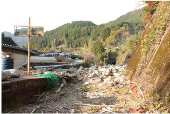
(b) Deposit of debris flow in the very vicinity of the station
