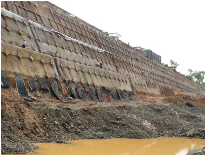
Fig. 2 Slope stabilization using grouted soil nail
