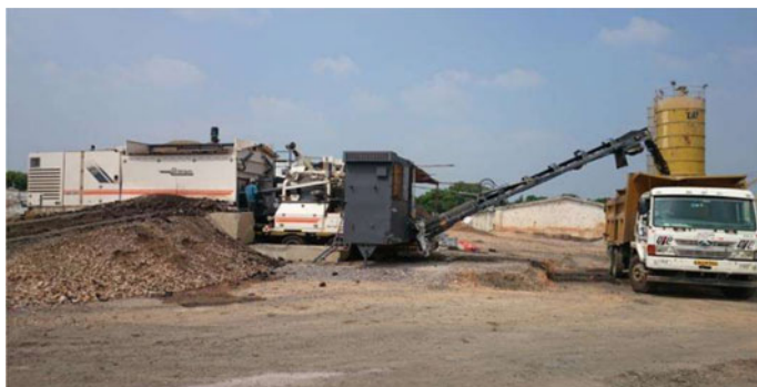
Fig. 13 Loading of RAP mix into dumpers
