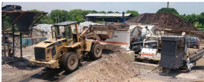
Fig. 12 Preparation of foam bitumen RAP in KMA plant
