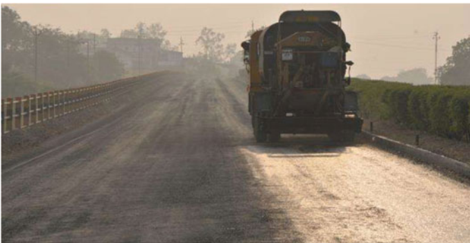
Fig. 17 Sealing of finished surface with Emulsion
