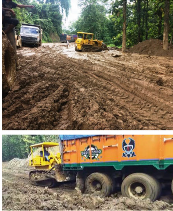
Fig. 17 NH-44 at Churaibari in July 2016 before rehabilitation
