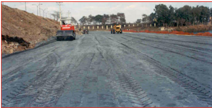
Fig. 5 Road embankment for Nizamuddin Bridge Project, Delhi
