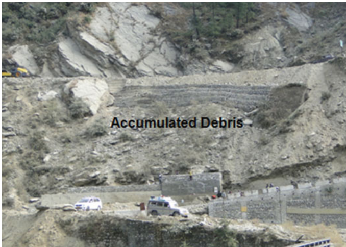
Fig. 13 Photograph accumulated debris at foot of the slide
