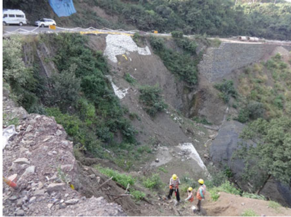
Fig. 8 Gabion foundation and dump on slope to receive RSS
