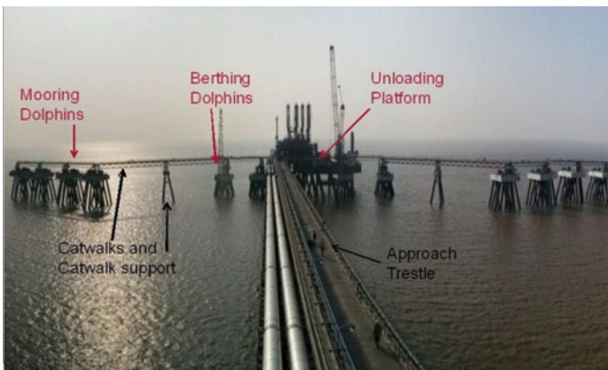
Fig. 1 Typical jetty structure
