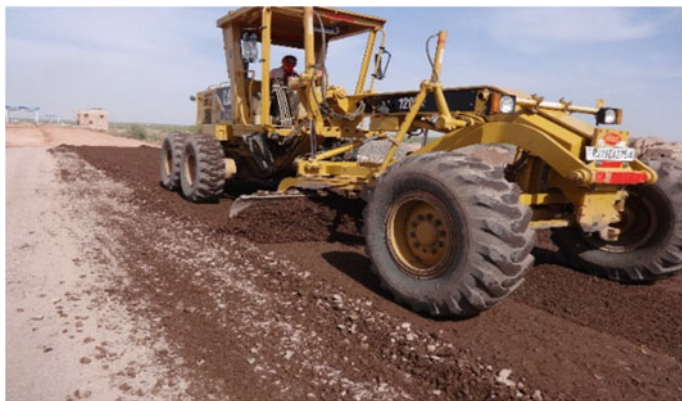
Fig. 7 Laying of CTSB
