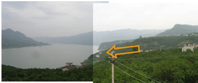
Fig. 9 Monitored slope in the Three Gorges Dam area in China
