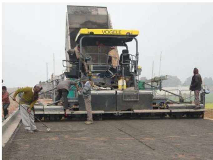
Fig. 14 Paving of foam bitumen-treated RAP layer using paver
