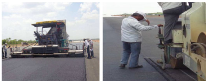
Fig. 5 Laying of DBM
