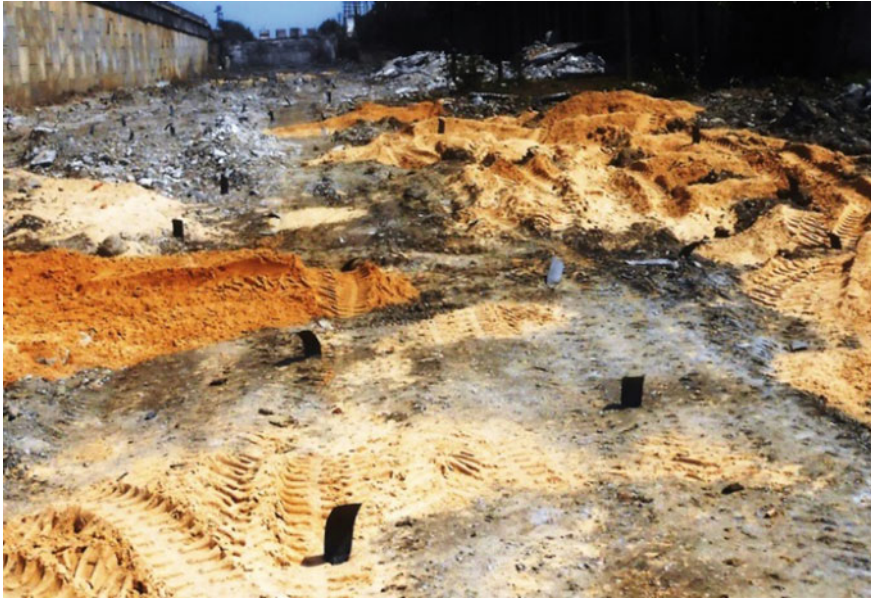
Fig. 8 PVDs for extension adjoining the existing structure
