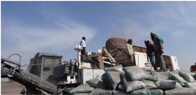
Fig. 6 Preparation of CTSB mix in KMA plant
