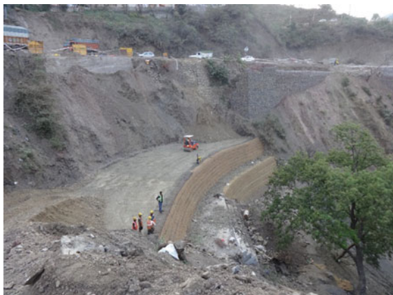
Fig. 10 RSS construction underway after the first berm
