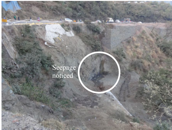
Fig. 9 Steady seepage is noticed on the hillside after clearing of slope face
