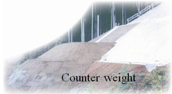
Fig. 23 Stabilization of an express motorway construction by counterweight
