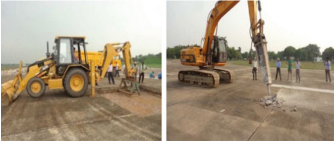
Fig. 4 Repair of broken slab
