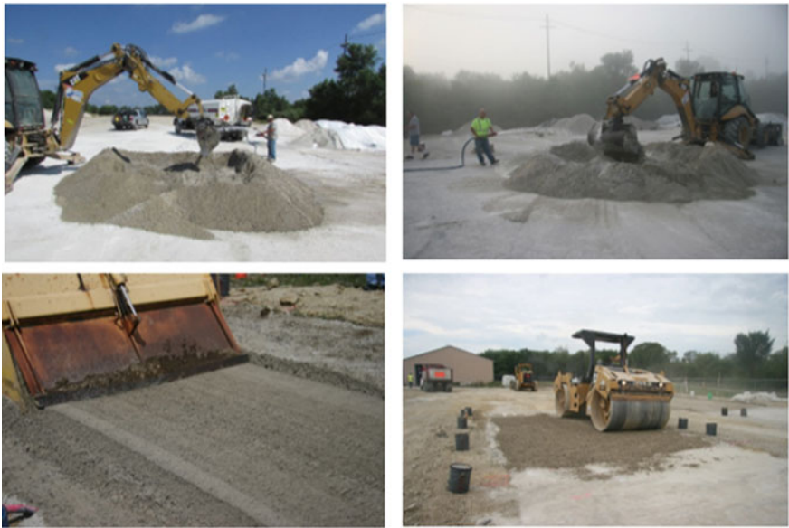
(b) Construction of cement and fly ash stabilized sections
