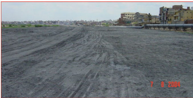
Fig. 9 Construction of Kalindi bypass
