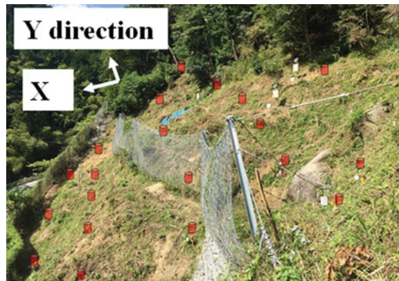
Fig. 27 Site of multi-point slope monitoring along a national highway
