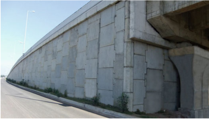
Fig. 10 Reinforced fly ash wall resting on fly ash-filled area
