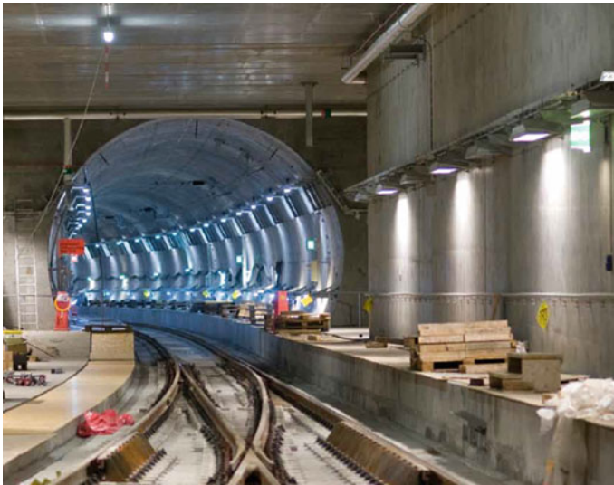
Fig. 2 Malmö City Tunnel Sweden (COWI 2009)
