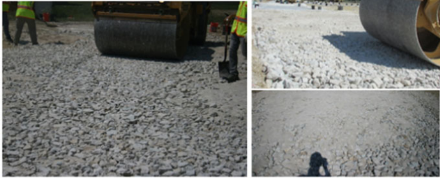
(a) Construction of C1S1 and C1S2 test sections
