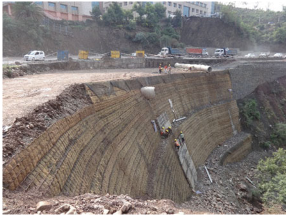
Fig. 12 Culverts to address the seepage water shown in Fig. 9
