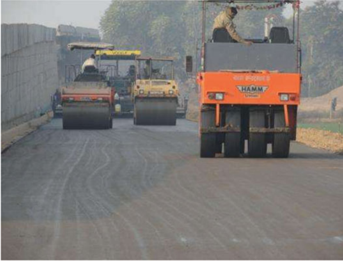
Fig. 15 Compaction operation in progress
