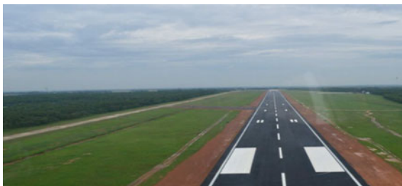
Fig. 11 Finished surface of runway
