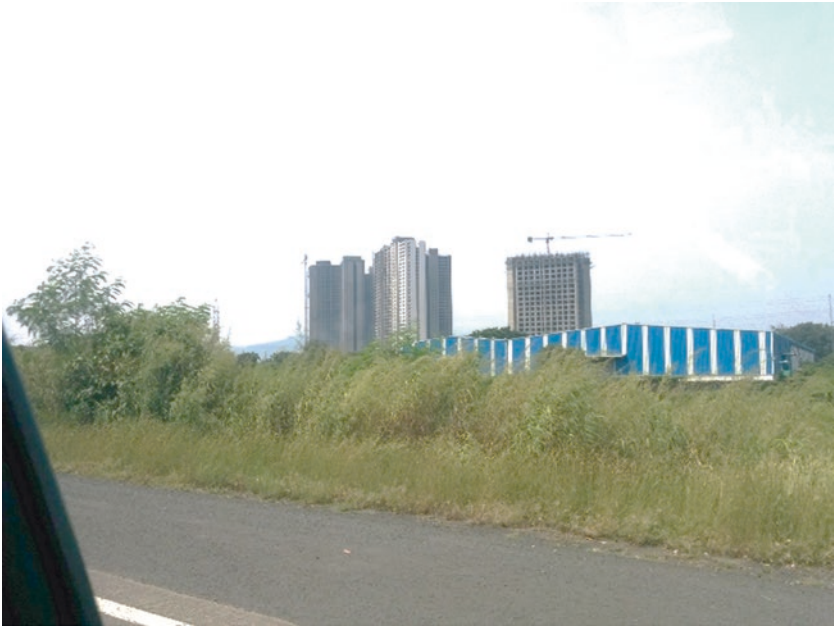
Fig. 10.3 Residential high-rise towers being built (Source: Photograph by author, 2016)
