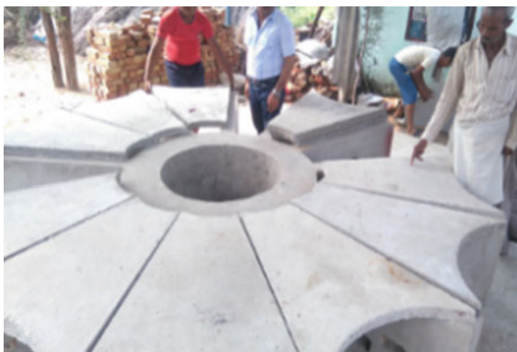
Fig. 27 Detachable shelves of raised platform
