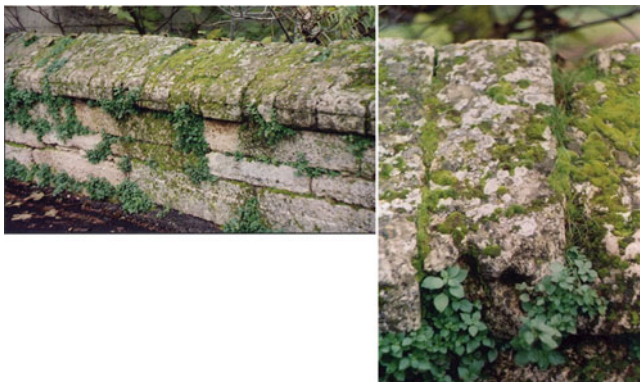
Fig. 10.14 Lichens (white-grey patches), mosses (green) and higher plants which are more apparent in winter with the increasing humidity on the calcareous garden walls in Edirne Beyazit Camii (mosque). (Photo by G. Küçükaya)
