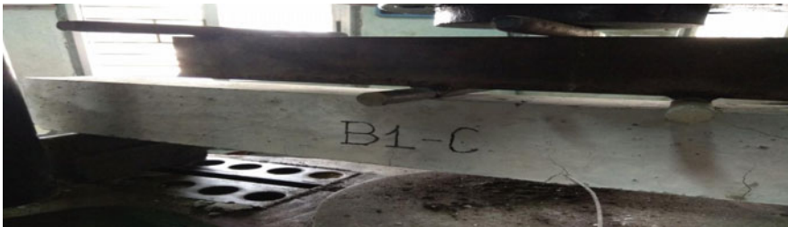
Fig. 7 Damaged beam 1 (C) with visible crack
