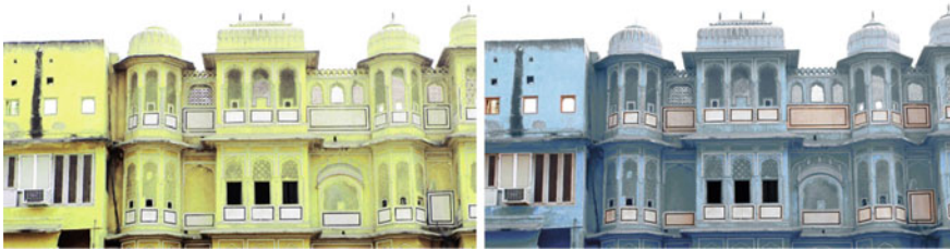
Fig. 32.5 Façade after changing colours. Source Author
