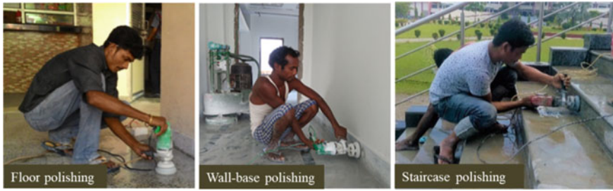
Fig. 47.1 Awkward postures adopted by the operators during polishing activities at different surfaces
