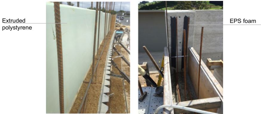
Fig. 8.5 Example of a curved reinforced wall with insulation, 2.5 \text{ m}^2 \text{ K/W} of thermal resistance, and a reinforced SRE beam with foam as an expansion joint (Photos Oliver Petrovic and Rodrigo Rocha 2014)
