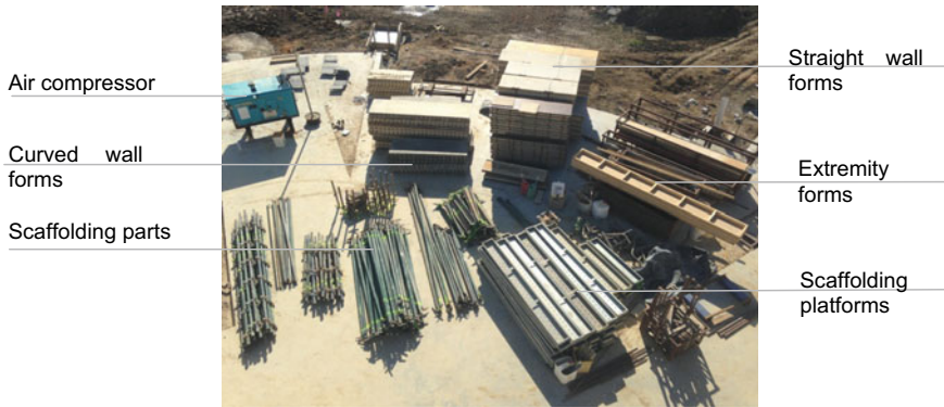
Fig. 8.1 Equipment used in the building process of the stabilized rammed earth (Photo Oliver Petrovic 2014)
