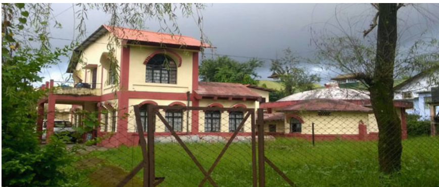
Fig. 13.14 1st SMB building in Shillong, constructed in 1995 and photographed in 2018
