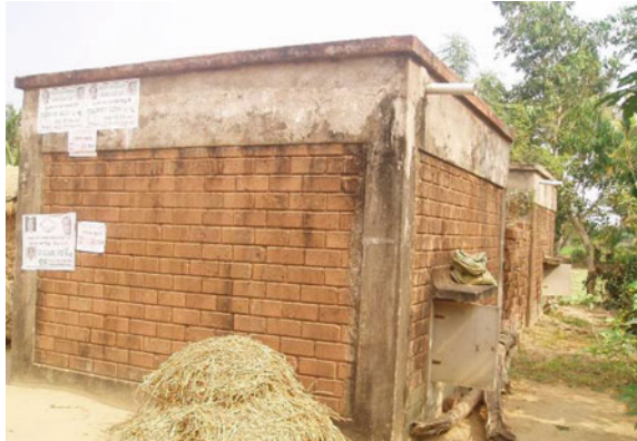
Fig. 13.11 Completed core house
