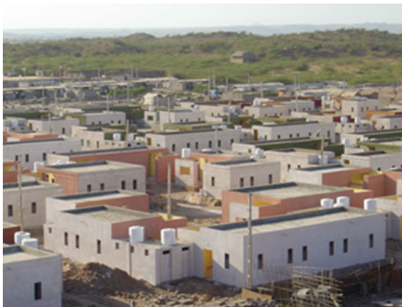
Fig. 20.8 200 CSRE houses with China clay waste
