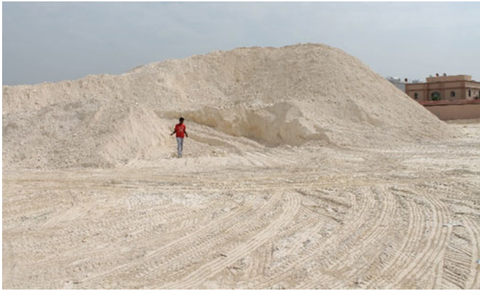
Fig. 11.6 A construction site with white marl in Saudi Arabia. Source Author, 2017
