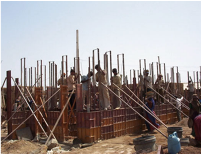
Fig. 20.3 Rectangular formwork
