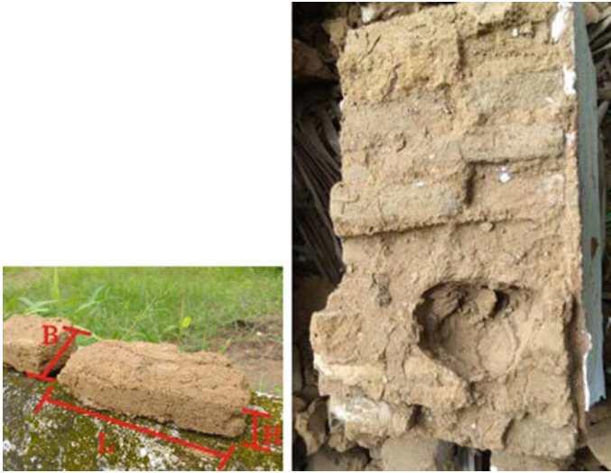
Fig. 37.5 Cross section of adobe wall
