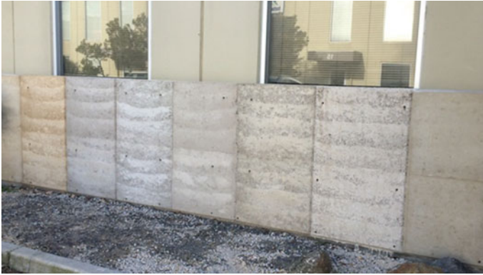
Fig. 8.4 Different SRE types on the forefront of the Olnee Constructions office ( Photo Rodrigo Rocha 2015)
