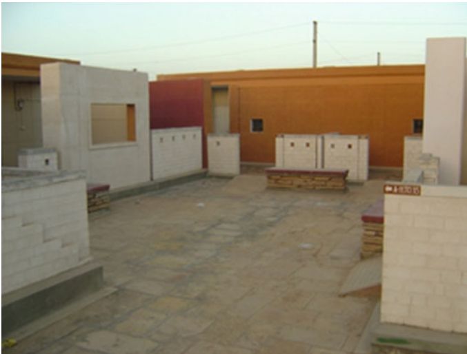
Fig. 20.6 A typical rectangular building with CSRE walls
