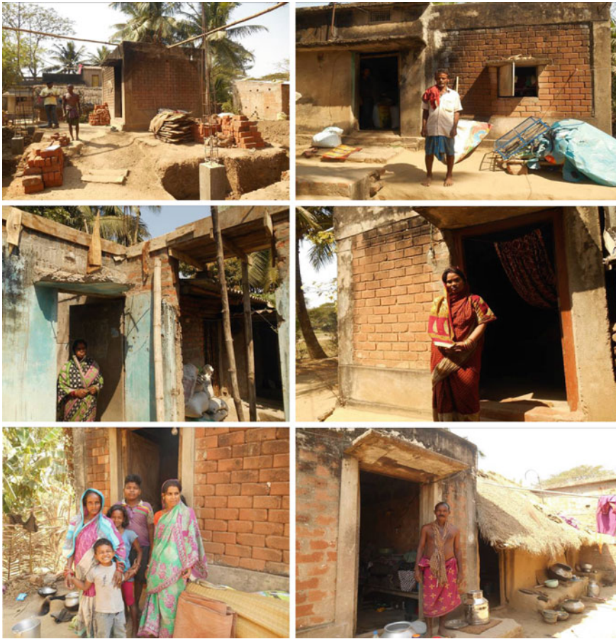
Fig. 13.13 Core houses in Patrapara village, Balikuda, Jagatsingpur, Odisha
