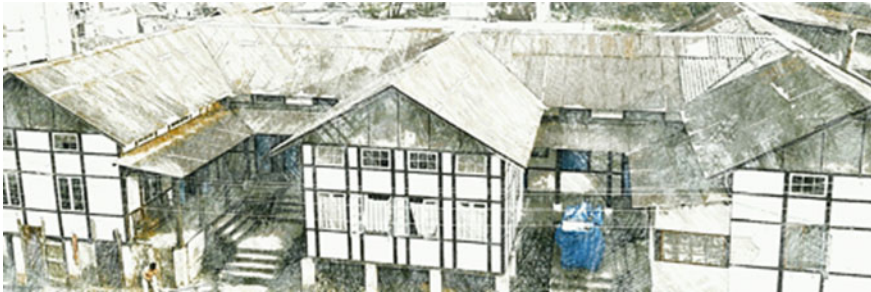
Fig. 36.1 Corrugated galvanized iron sheet roofing of Integrated Craft Complex of Craft Based Resource Centre and Material Bank, Shillong
