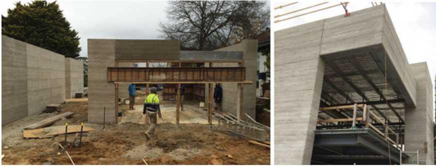
Fig. 8.9 SRE building process over T-shaped steel beams (Photos Rodrigo Rocha 2015)
