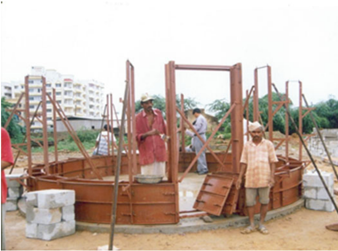
Fig. 20.2 Circular formwork
