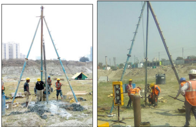
Fig. 18.8 Boreholes and pressure meter tests in progress
