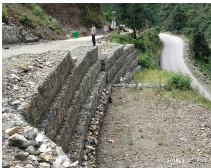
Fig. 19.18 Retention works at hairpin bend at Birahi site
