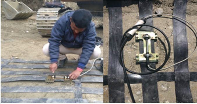
Fig. 19.21 Implementation of strain gauge at the site
