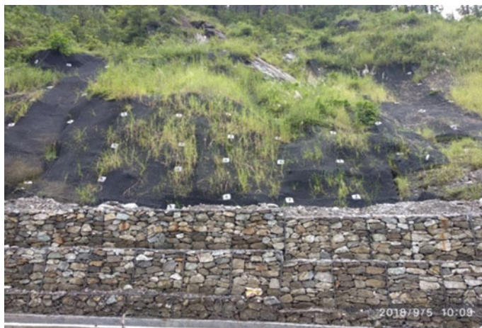
Fig..19.17 Rockfall mitigation and erosion control at Birahi
