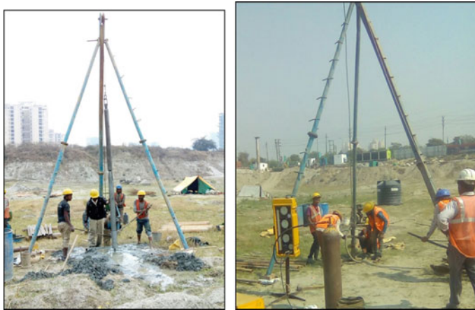
Fig. 18.8 Boreholes and pressure meter tests in progress
